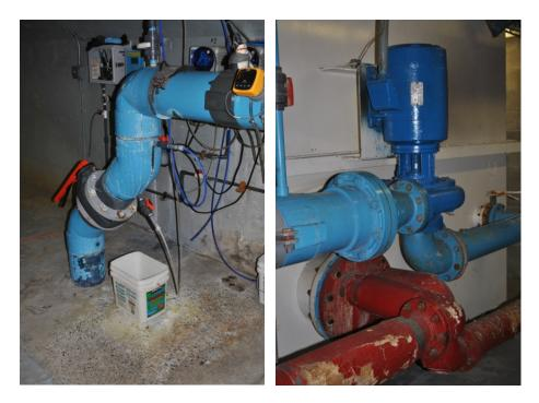
Replace all pool water plumbing in the mechanical room including valves, flow meter, reducer, bypass, etc., many of the valves are inoperable and broken, current plumbing has weakened spots that are small leaks. Bring plumbing up to code and install better isolation valves for easier maintenance in the future.
