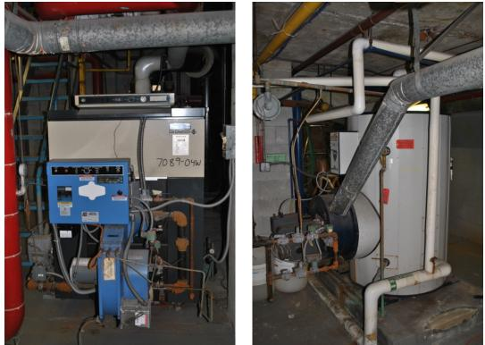
Replace domestic hot water tank with new high efficiency condensing boilers. The existing boiler is on its last year of rated life expectancy.
